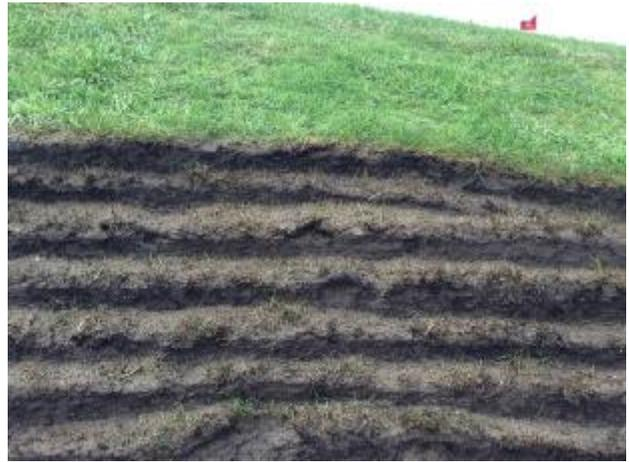
Figure 2: The quality of revet turfs is good. It is pleasing to see the finished article with the grass growth burnt off to present a clean face.
